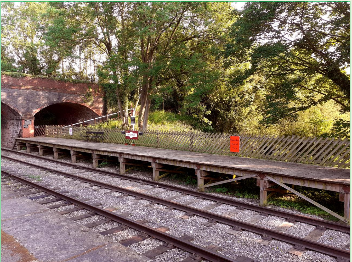
Shottle Platform 2 on completion by the Trust, Spring 2023
