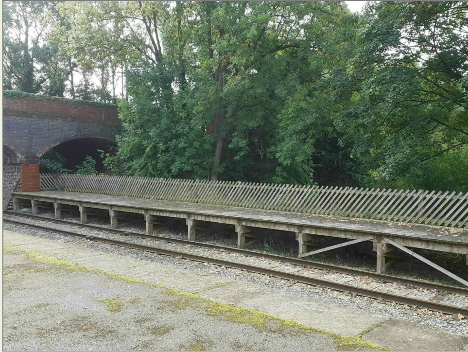
Shottle Platform 2, five years after construction
